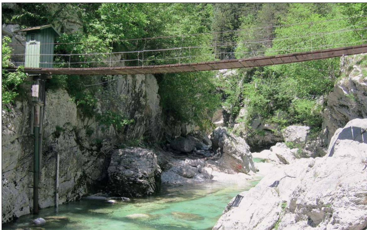
Vodomerna postaja ob reki Učja v kraju Žaga. (foto: Peter Frantar) Surface water gauging station on the river Učja in Žaga. (photo: Peter Frantar)
