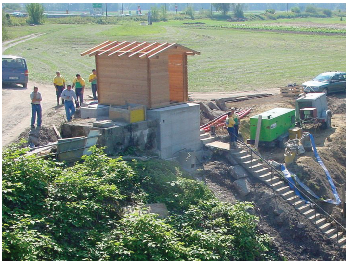
Obnova in posodobitev vodomerne postaje Šentjakob na Savi. (foto: Marko Burger, 17. september 2003) Reconstruction of gauging station at Šentjakob on the Sava River. (photo: Marko Burger, 17 September 2003)
